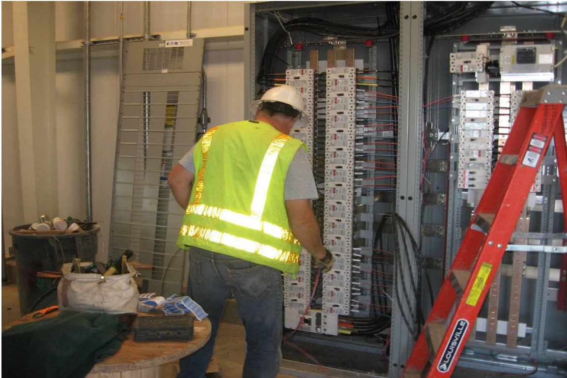
Subcontractor Central Sierra landing conductors in electrical distribution panel DCA.
