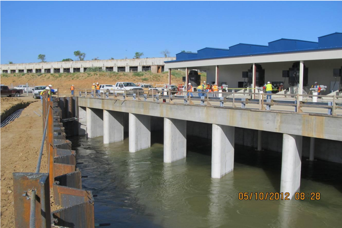
Start of pump test water flow in canal transition.
