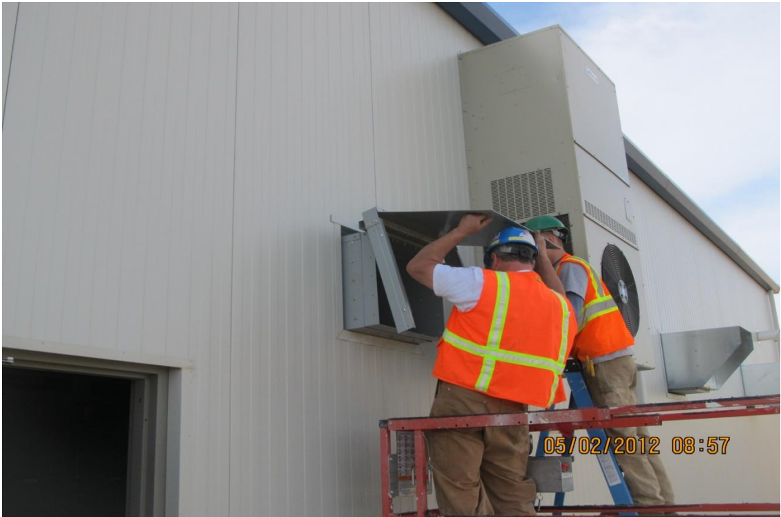
Subcontractor Central Sierra Electric installing the Arc Flash plenum ducting.
